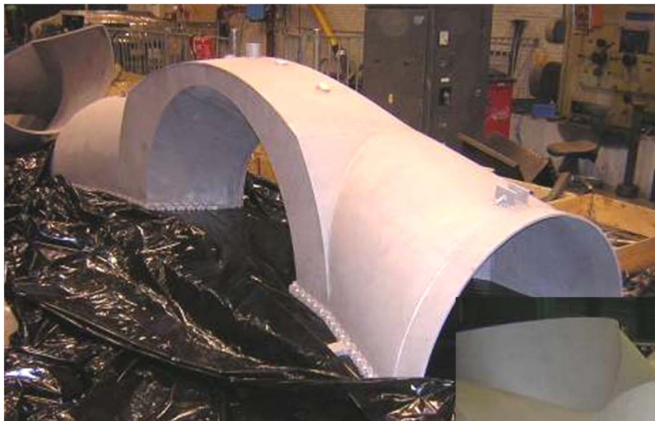
New & repair Inner casing
