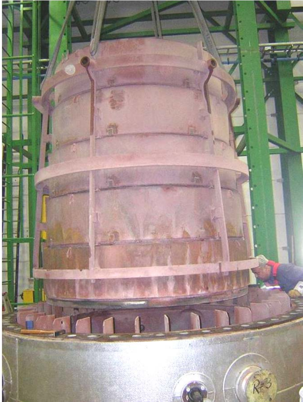
disassembly upper combustion chamber
